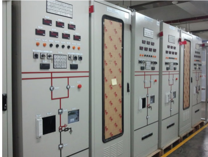
Gambar 2.5. Gambar Panel Trasn misi Trafo Bay 150kV / 20kV(Aslimeri, 2008)
